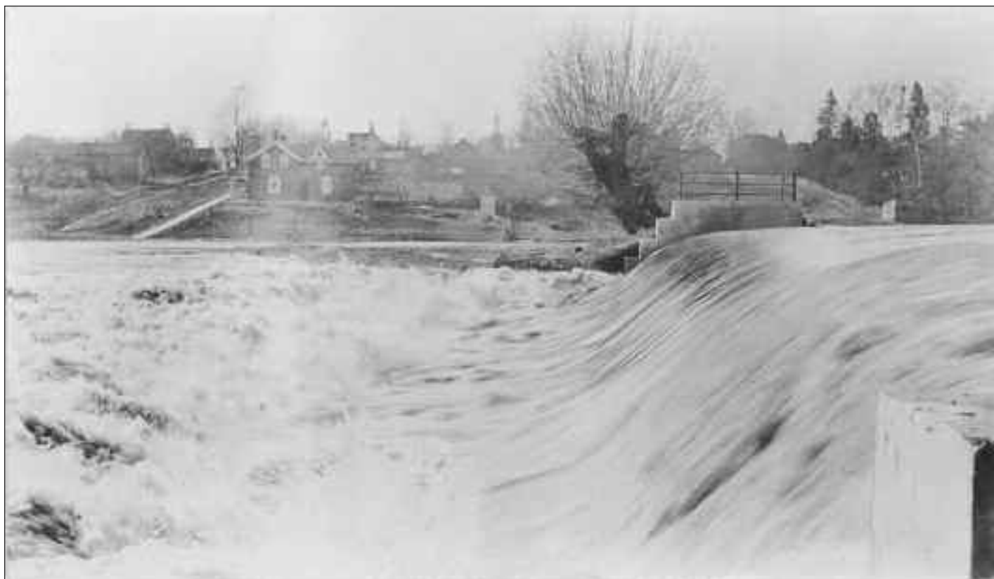
0027 A photo of the Thames River roaring over the flood wall and through Mitchell's broken dam in April 1912. The flood was caused by a spring thaw more rapid than usual. This photo was taken from the river's eastern shore, near the sluice gate of the dam.
