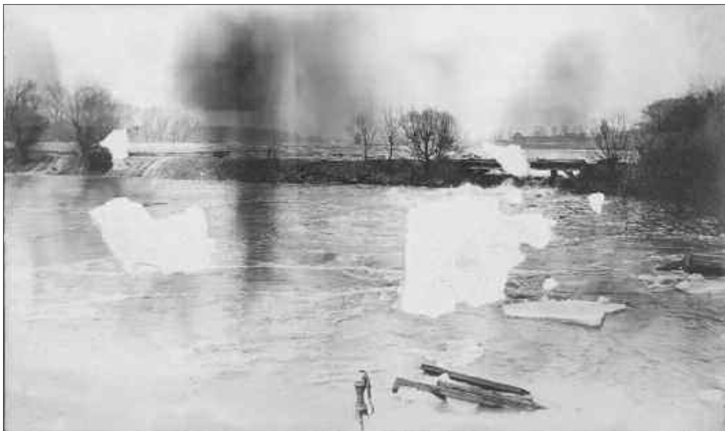
0023 A damaged photo of the Thames River and ice flowing over the flood wall and through Mitchell's broken dam in April 1912. The flood was caused by a spring thaw more rapid than usual. It resulted in an upstream ice-jam breaking through a protective log boom. This photo was taken from the river's eastern shore, downstream of the dam.
