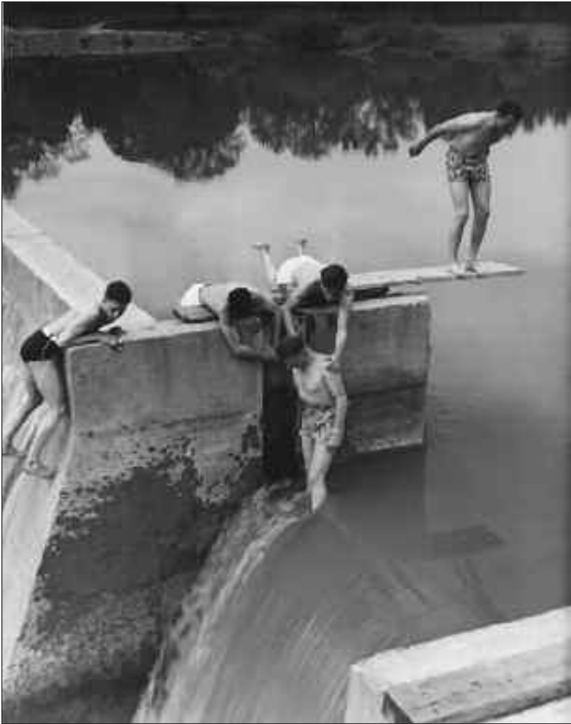
0031 Five unidentified young men play on the dam and in the Thames River in the 1950s. This dam, the second to help control the flow of the Thames through Mitchell, was replaced by a more substantial structure in 1962-63.
