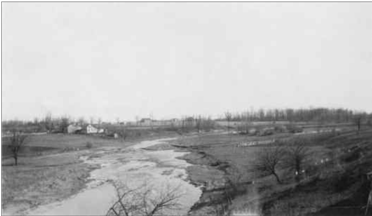
0022 A southerly view of the Thames River, downstream from the Toronto Street bridge, where it is joined by Whirl Creek, flowing from the east.
