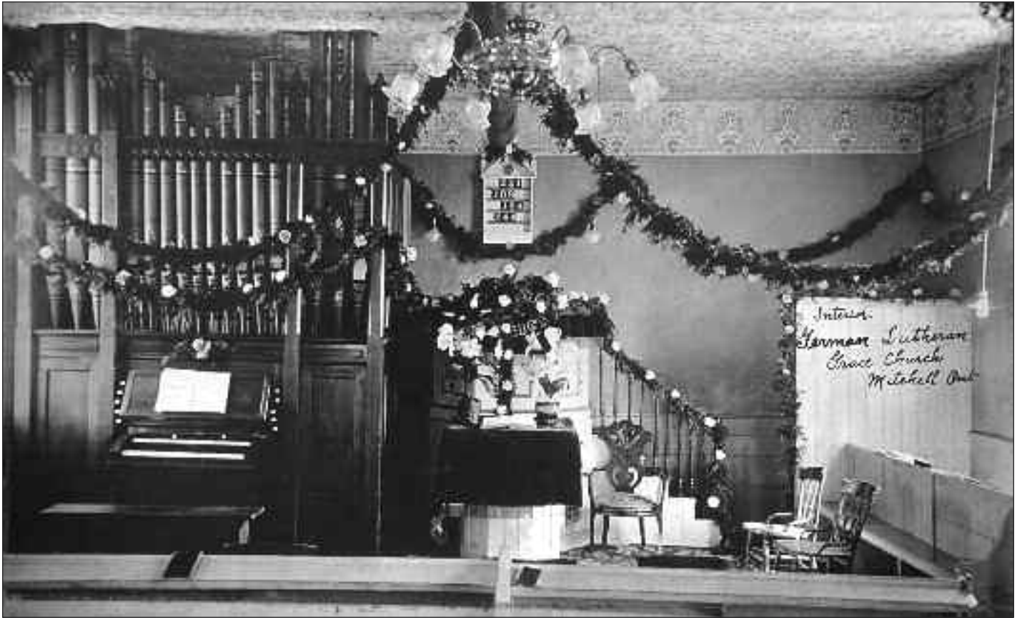
0511 A view of the sanctuary in Grace Lutheran Church, which was built in 1914 on the northwest corner of St. David and Quebec streets.
