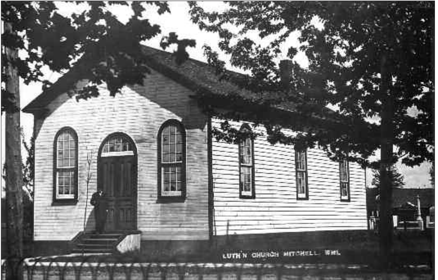
0510 This is the first Grace Lutheran Church in Mitchell. It was built on Highway 23, north of the town, where the Lutheran cemetery remains today. It was in use until 1914.
