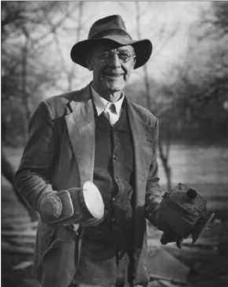
1508 Dave Eizerman (1887-1957), a member of the Mitchell Lions Club, worked without fee in overseeing the club's construction of a municipal swimming pool on Blenheim Street, just east of Nelson Street, in 1948-49.
