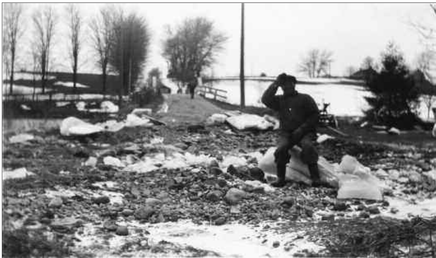
5506 Wilson Brown sits on a chunk of ice on a washed-out part of the road near the Motherwell bridge in Fullarton Township on April 8, 1947. The ice deposits came from floodwaters of the Thames River, which took out much of the road. About 100 tons of stone were required to rebuild the road before it could be surfaced with gravel.
