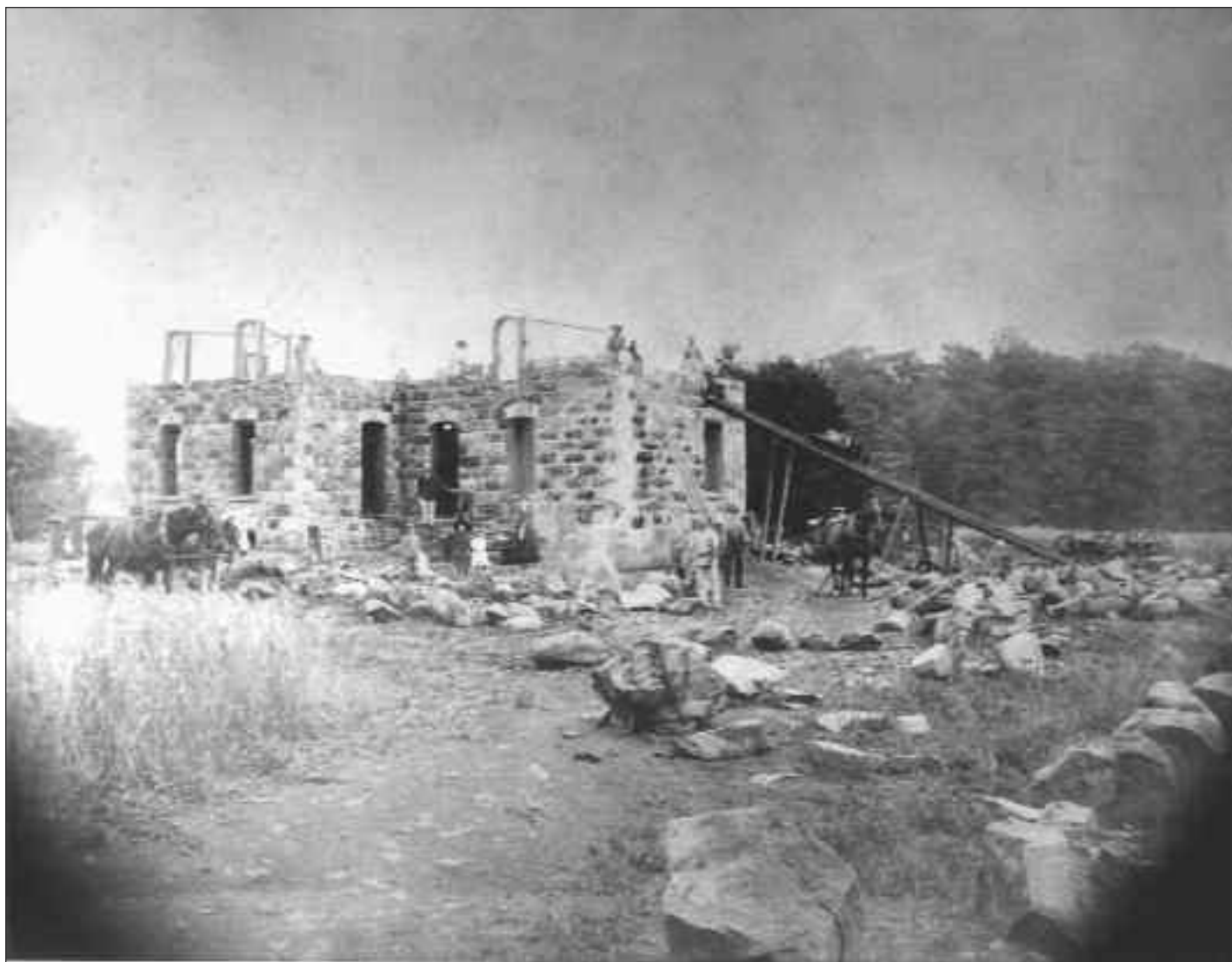
5507 Construction of a stone house near St. Pauls in Downie Township. Close to the near corner, men are using sledgehammers to break up stones. Other workers use a winch to pull a small wheeled car full of stones, up a ramp. Some of the other men in the photo, as well as the women and children, are likely friends or relatives of the workers or the owners of the house.
