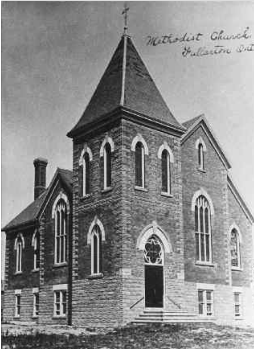
5515 The Methodist Church in the village of Fullarton, Fullarton Township, soon after it was built in 1908. (4)
